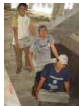
The seminarians are experiencing sweat and tiredness in construction work.
